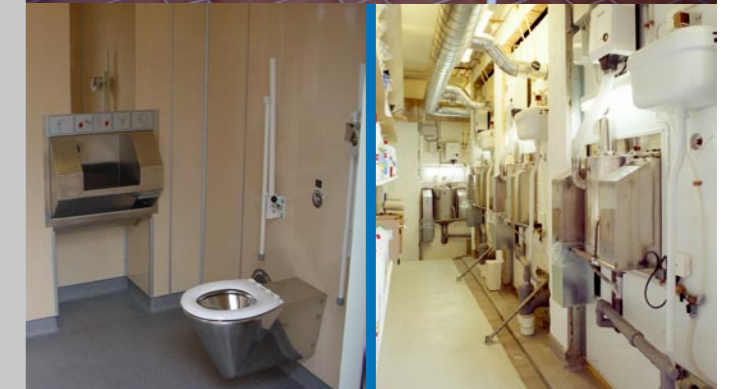
Cubicle easily accessible
