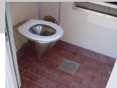
Standard size cubicle with tile flooring.
